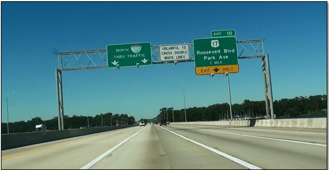
Figure 4-9 Sign Gantry Prior to Bridge Exit
