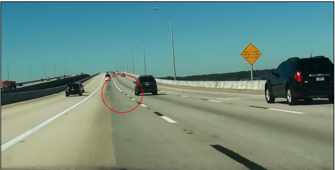
Figure 4-4 Solid Lane Striping in 2nd Lane and First Side Mounted Warning Sign
