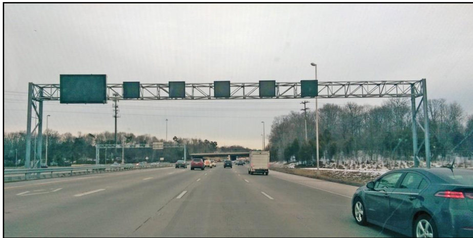
Figure 7-4 I-66 Active Traffic Management System. Fairfax, Virginia
